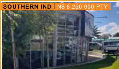
SOUTHERN IND | N$ 8 250 000 PTY HYPER MOTOR CITY Levy N$ 3 000 per month. +/- 450m 2 . Large Showroom Area, Kitchenette, WC, Shaded Parking.
