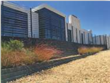
Extending land for building
