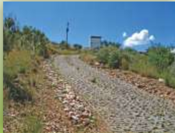
Rustic and permeable road erosion control
